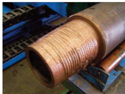
Too much thread compound
